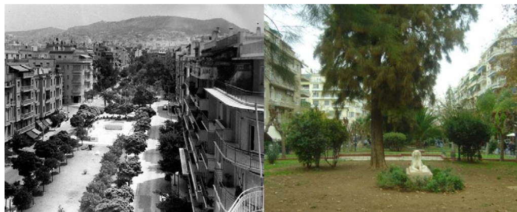
Fig. 1. (left) Panoramic view of Fokionos Negri Street and Ano(Upper)Kypseli from the height of Ioannou Drosopoulou Street (1964) © Billy Files (source: http://vintage-files.blogspot.com/ ) (right) View of the linear park of Fokionos Negri in the 21st century (source: https://commons.wikimedia.org/wiki/File:Fokionos_Negri_View.JPG )
