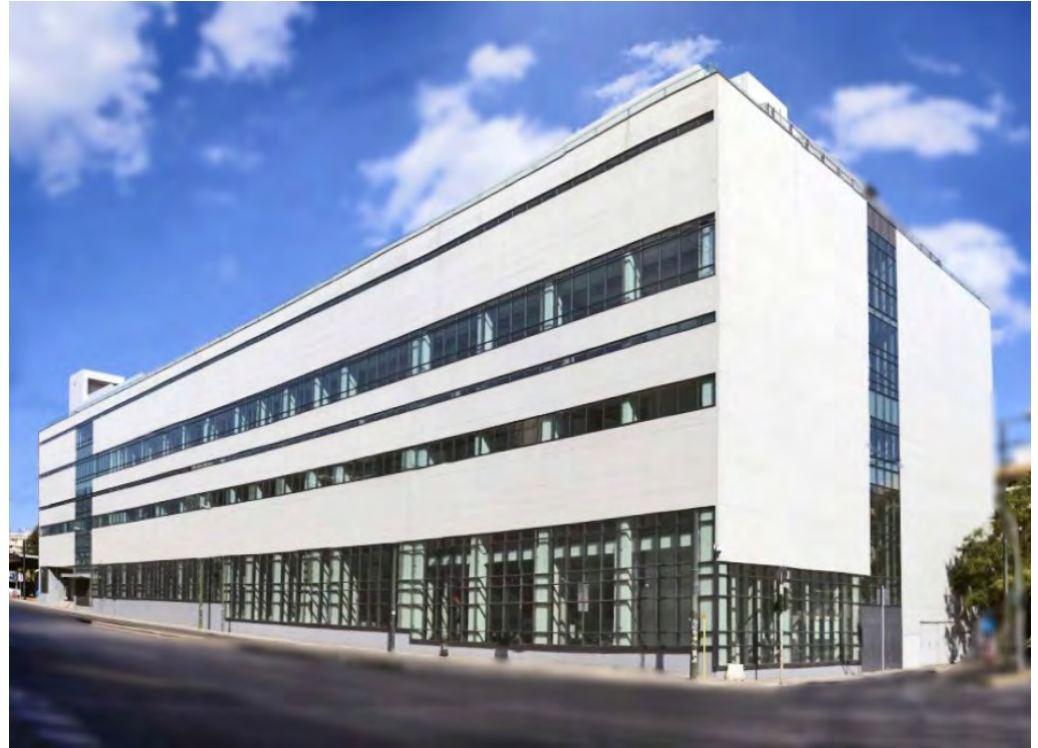
Figure 2 – Sygrou Avenue current façade view of the adaptively reused iconic FIX Brewery to house the EMST (2020).
