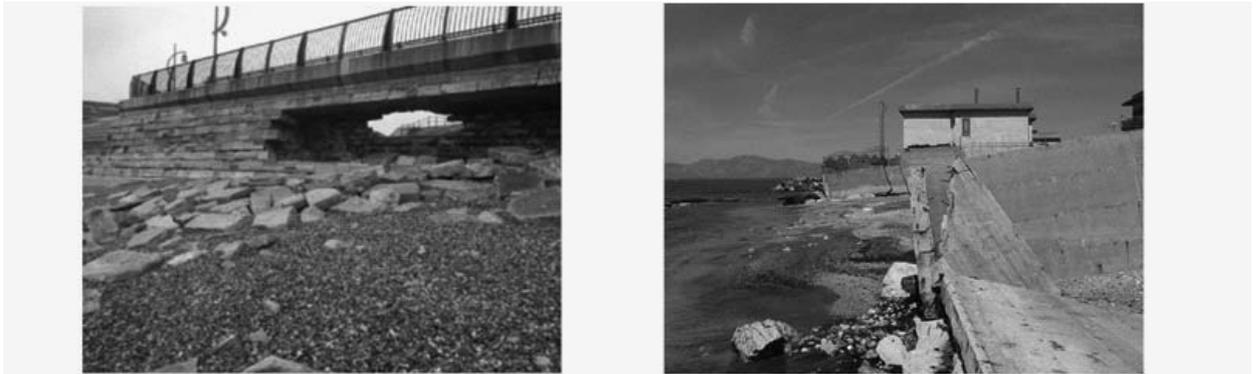
Figure 1 – Collapse of coastal defences in Portsmouth (left) and coastal erosion and flooding consequences on a shoreline house in Litorale Domitio (right)
